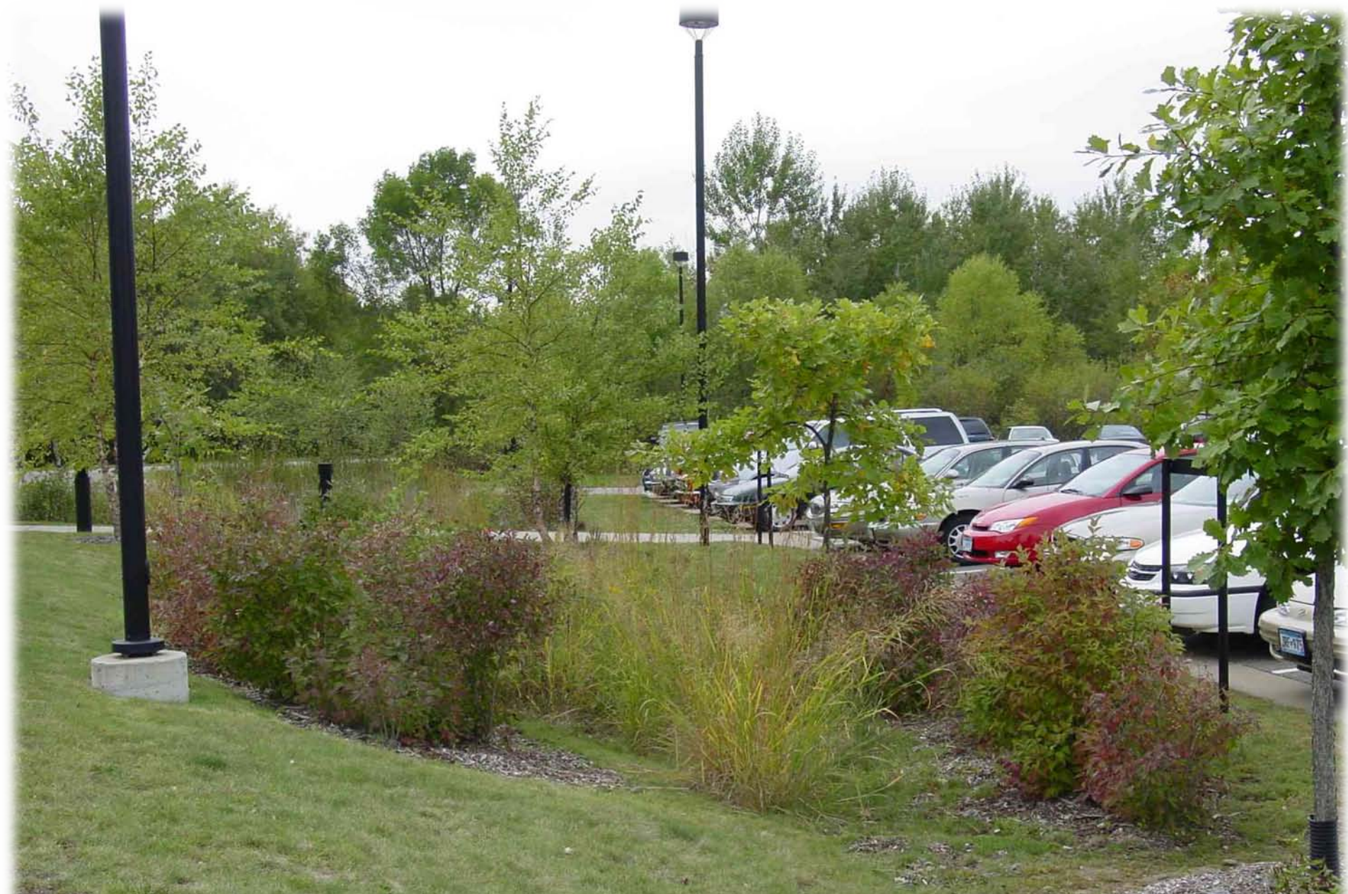
A Rain Garden to Capture Runoff from the Parking Lot and from the slope.
